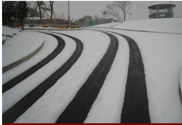
Heatizon Constant Wattage MI Cable
