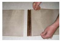
Step 2: Flatten the connection by crimping or compressing the splice plate down on top of both pieces of ZMesh using a short length of 2x4 stud or by tapping gently with a hammer or rubber mallet.
