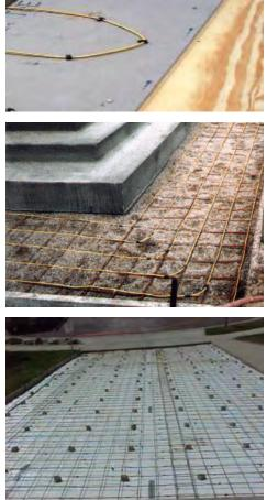
f. If a temperature/moisture sensor such as the Heatizon M331 or M336 is to be installed in the concrete, mud bed, mortar, or sand bed, it must be in place prior to covering. See the sensor installation instructions for details.
