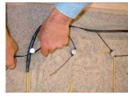
**Step 7.** Cover Tuff Cable with ½" of sand. Make certain that the Tuff Cable is surrounded by sand. Never allow Tuff Cable to directly touch itself or the insulation. Always make certain that some sand gets between the bottom of the Tuff Cable and the insulation. Great care must be taken to avoid damage to the Tuff Cable.
