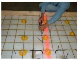
8. Complete tying of any Tuff Cable, and trim any untrimmed wire ties.
