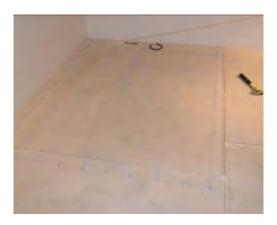
**3.** If Tuff Cable is being installed on wood subfloor, mark adjacent runs of element on the floor with appropriate spacing, usually 6 to 8 inches (but in some cases, may be 4, 10 or 12 inches). Verify specific spacing requirements for your installation with those in your heat loss calculation for space heating.
