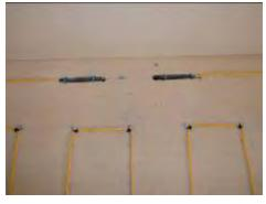
Tuff Cable under hardwood in lightweight concrete.
